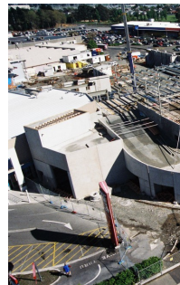
Aerial photograph of the main contractor's site.
