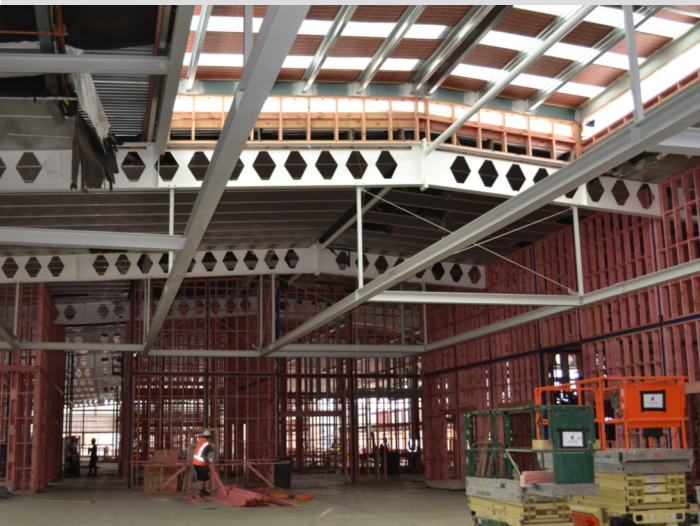
Pictured above, the link between 901 and 902 looking towards Broadway. Below a raised skylight in 903 illuminates existing castellated beams that have been preserved. Right, strengthening the walls of 904 with steel columns and bracing.
