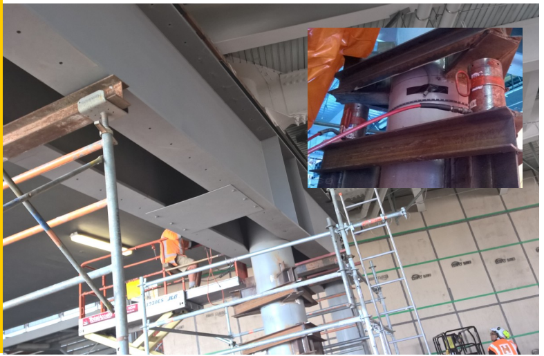
The retro-fitting of 32 Oxford Street with Star Seismic BRBs (Buckling-Restrained Braces)
