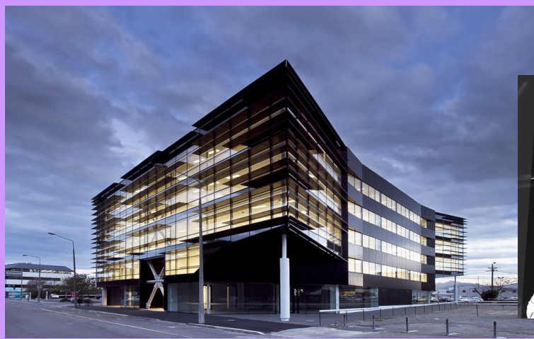
The retro-fitting of 32 Oxford Street with Star Seismic BRBs (Buckling-Restrained Braces)
