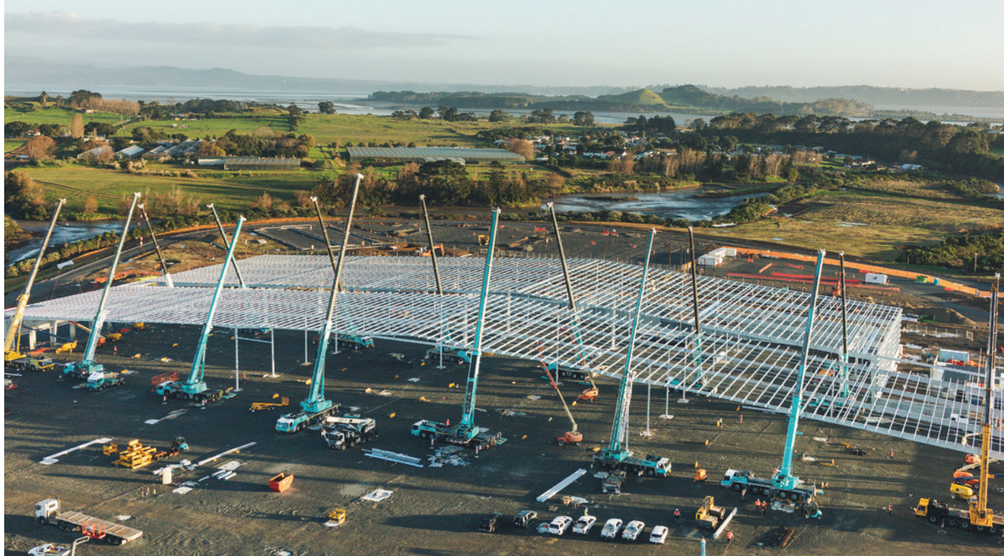
Below: A massive simultaneous steel 'lift' using 16 cranes at the Foodstuffs North Island Distribution Centre was no mean feat for D&H Steel.
