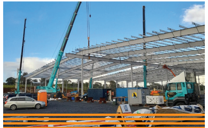
Above: 24 Custom Welded Beam portals provide the largest possible clear-span envelope, so the fitout won't be impeded by the supporting structure.
