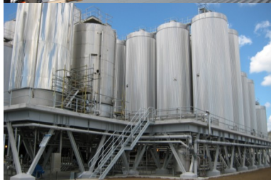
Below: Each of the 58 vessels making up the tank farm weighs 250 tonnes fully loaded. The complexity of the angles of the supporting structure demanded the best of D&H design and steel detailing.
