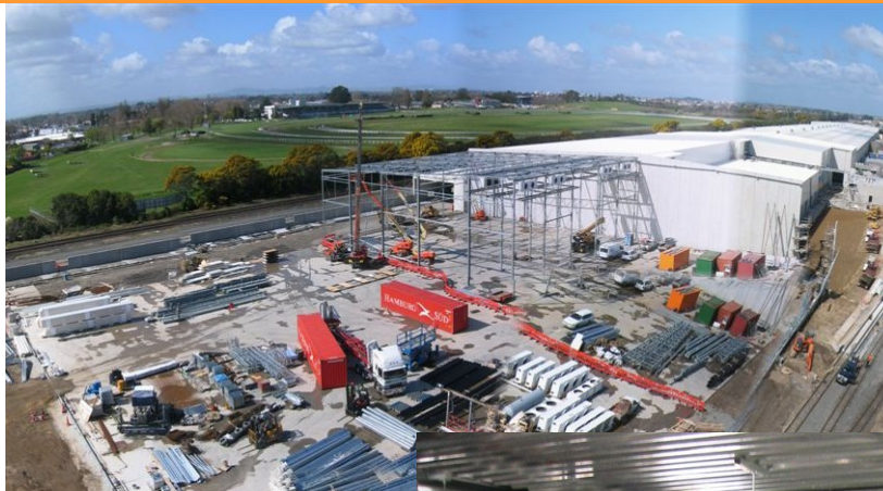
Right: Fonterra's new plant at Te Rapa, Hamilton — large freezer spaces at -8^{\circ}\text{C} .
