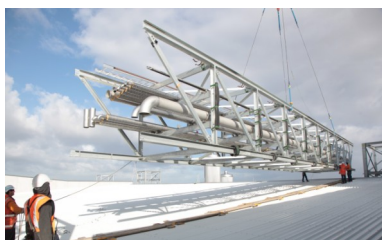
The 20,000m 2 Packaging Hall is 150m wide. It has 33 trusses, two spine trusses and very few columns.
